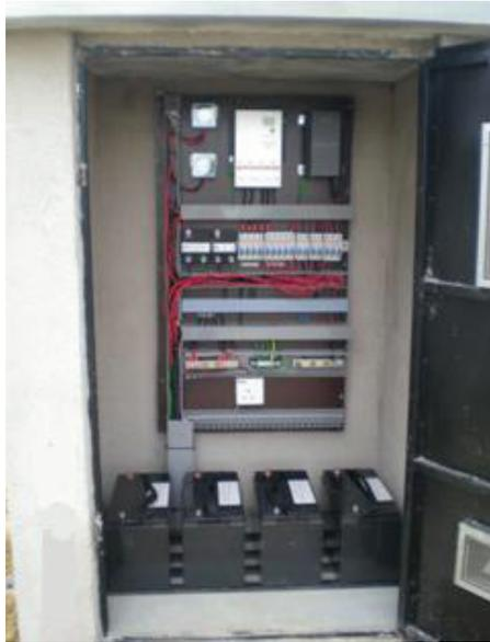
**FIGURE 7** Housing for Batteries and Balance-of-system Components
